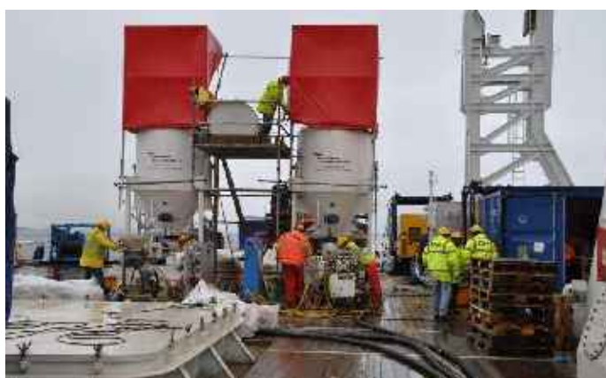
Figure 16 – Atelier de cimentation offshore (source DONG Energy)
